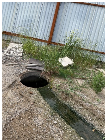
Photo 6: Manhole without cover
